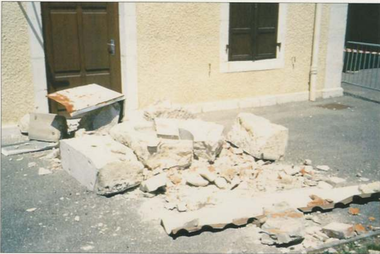
Plate 2. Earthquake damage in Metz-Tessy from the Annecy earthquake 15 July 1996 00:13 UTC, magnitude 5.3 ML. (Photograph supplied by Francois Thouvenot, LGIT - Observatoire de Grenoble, Grenoble)
